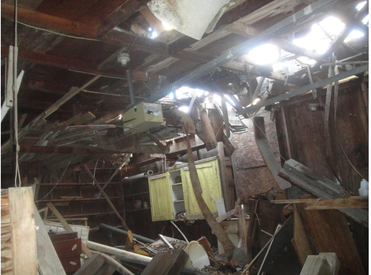
Photo 13 – View of collapsed garage ceiling.
