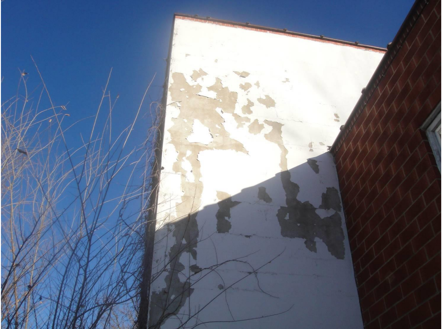
Photo 25 – Deteriorated siding material, 110 W. Main Street.
